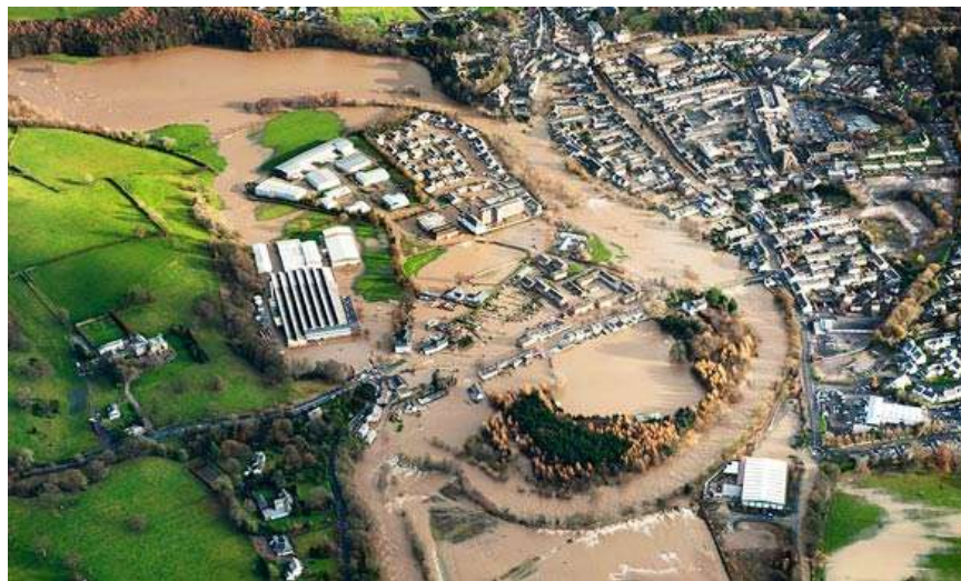
Figure 30 Flood costs in Cumbria are not a hypothetical risk scenario; they are very real and very expensive. The flooding of Cockermouth in this image was an enormous human and financial disaster for Cumbria.
